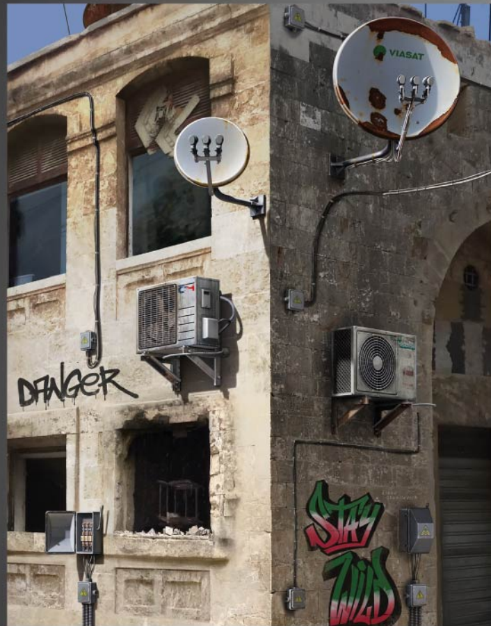
35638 AIR CONDITIONERS & SATELLITE DISHES
